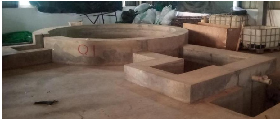
Figure 2. Circular concrete tanks that can be used in semi-natural spawning of L.victorianus
