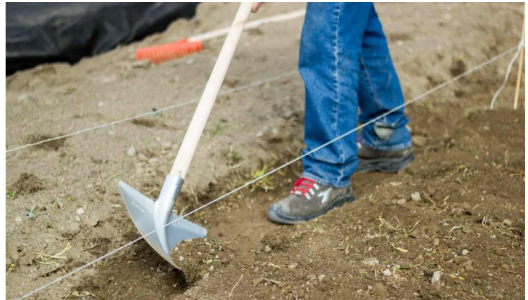
Prepared soil for mulching operation
