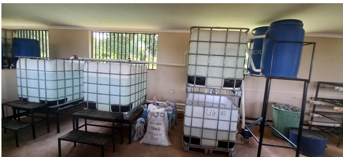
Figure 22: A cost-effective RAS unit that uses locally available biomedica and is solar powered
