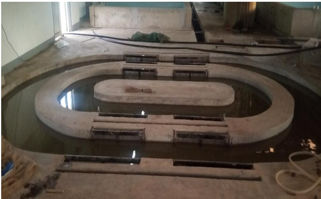
Figure 39. The hatching system was designed for cyprinids, where eggs in this trial were inoculated for incubation and subsequent hatching.
