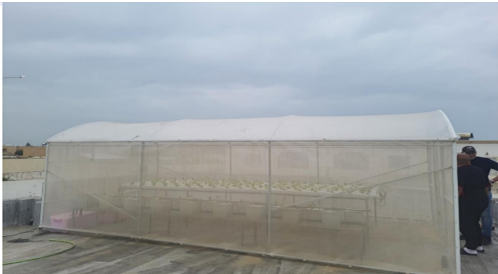
Figure 5 Greenhouse on a rooftop in Tunisia (Credit Jamai D.)
