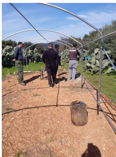
Figure 7 Soil levelling and iron frame installation (Credit Jamaï D.)
