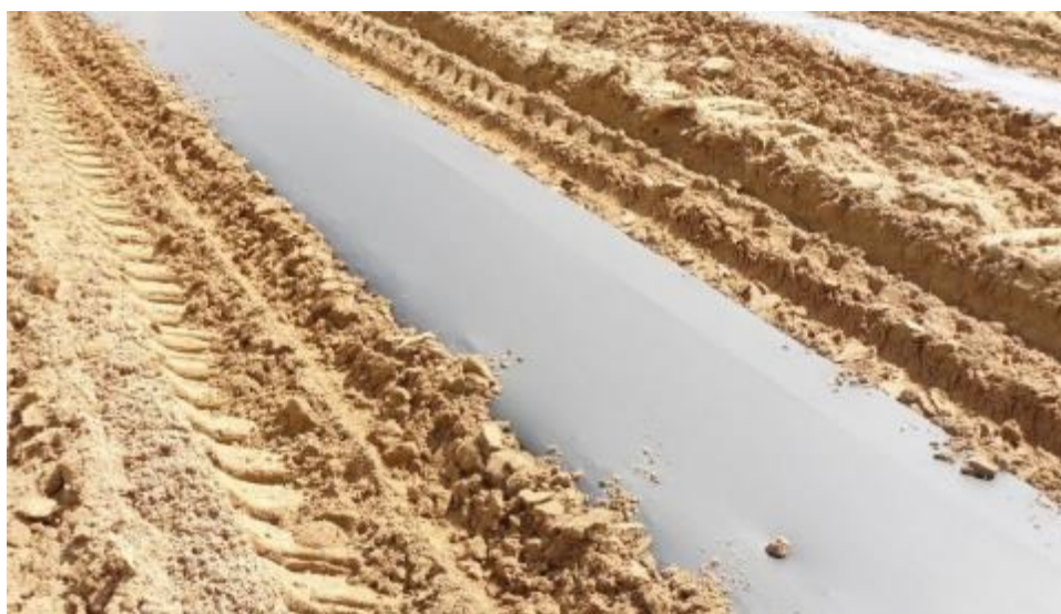
Figure 19: Layed mulch film
